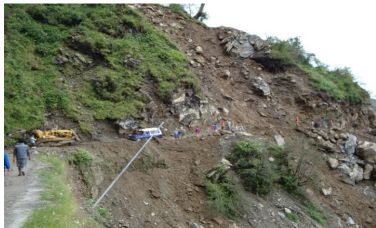
Fig. 1: Various landslides in Sikkim
